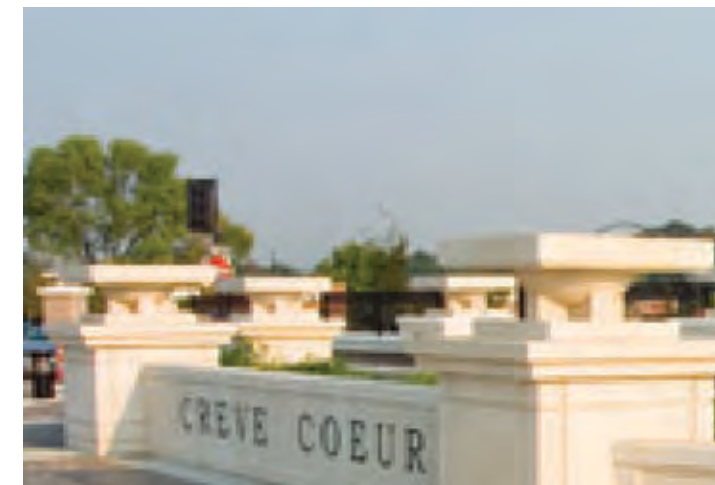
New Olive Boulevard bridge over I-270
